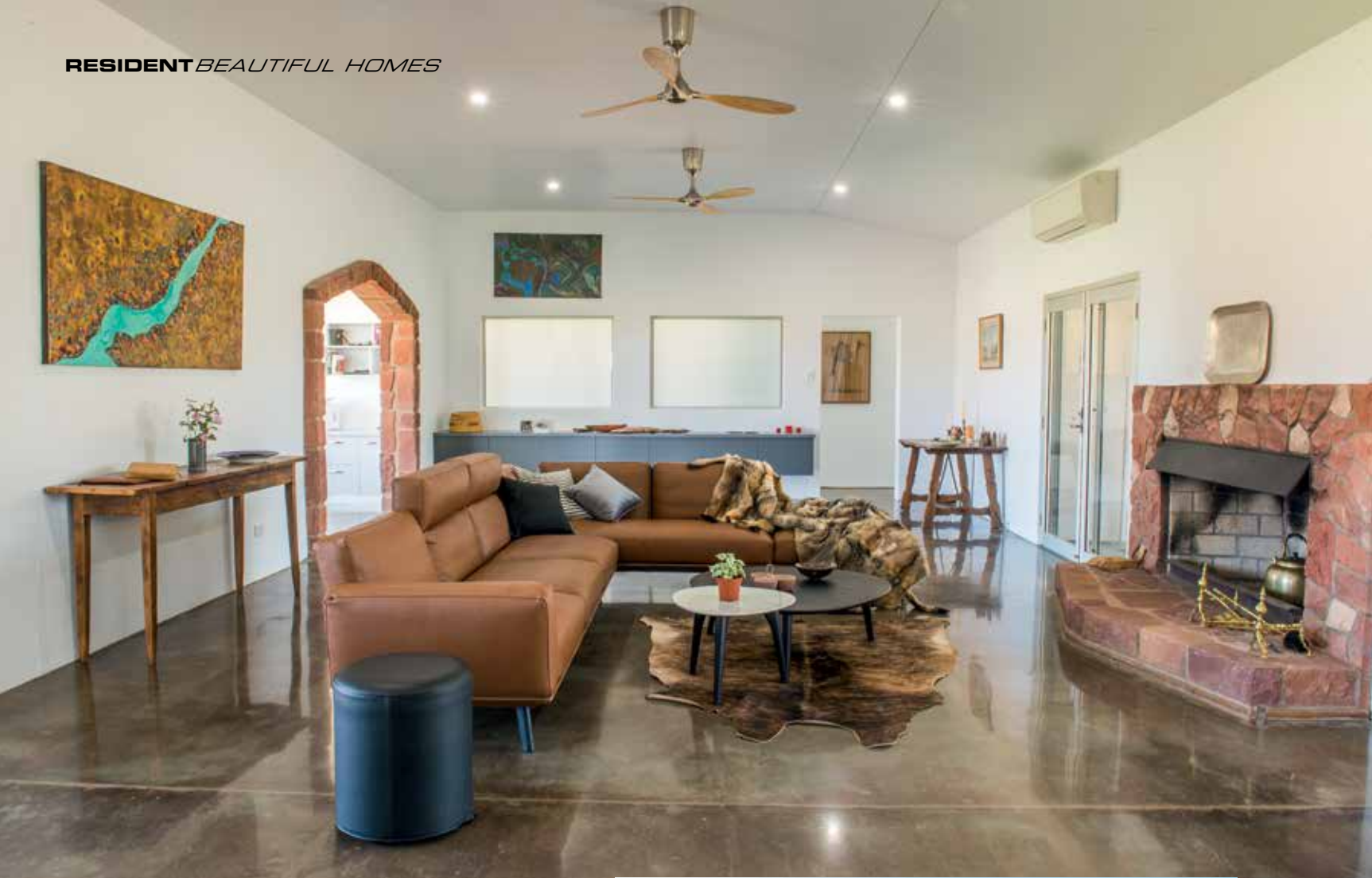
The flooring is polished concrete, made using sand from the local creek containing all sorts of rocks and pebbles in varying shapes, colours and sizes. Brad spent six weeks grinding and polishing to get the very best result.
