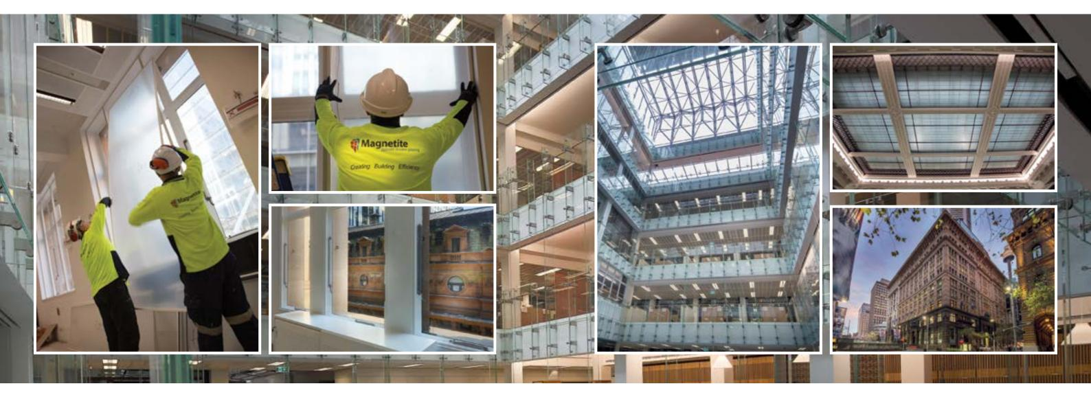
Magnetite (Australia) Pty Ltd was contracted to retrofit double glazing to 362 windows in the 5 Martin Place Redevelopment project. Magnetite manufactures and installs a secondary window system designed to reduce noise and reduce energy consumption.
